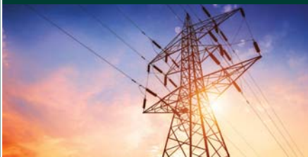
Electric Generation and Transmission
