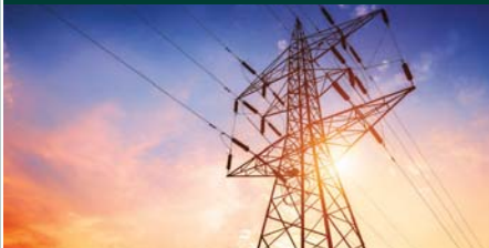
Electric Generation and Transmission
