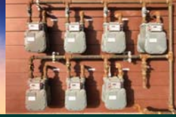
Natural Gas Transmission
