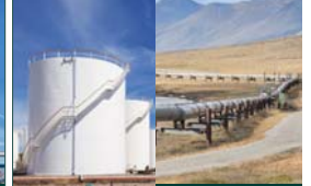
Transportation, processing, and storage of crude oil, natural gas, and products
