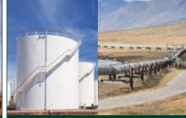
Transportation, processing, and storage of crude oil, natural gas, and products
