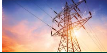
Electric Generation and Transmission
